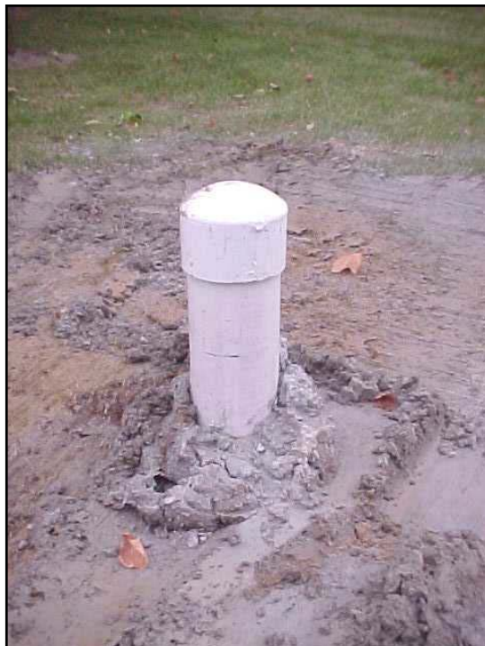
Temporary well cap - installed between well drilling and pump hook-up
